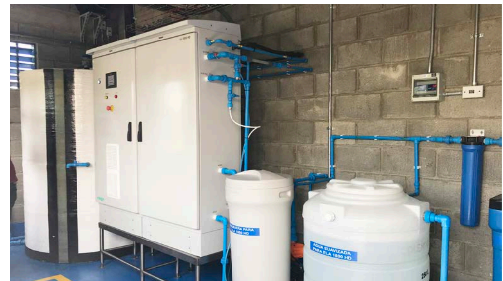
Enviolyte ela1800HD set for 5000ppm for public water treatment
